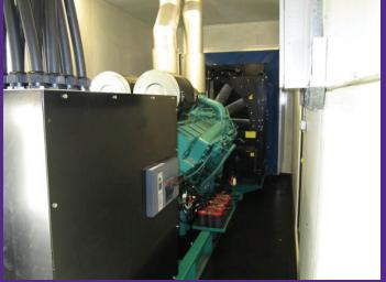
the system is menu driven and simple to follow with different levels of access available as appropriate to operator capability of engineer modifications. An additional benefit of the system is that all information available from the set mounted panel is mimicked to the Master Panel which in this instance was located in the LV Switch room; this allowed all relevant information on generator and switchboard status to be available in the same place.
